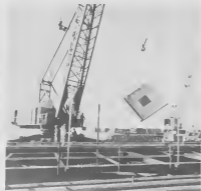
One of the two-ton concrete slabs is carefully lifted from the walkway to permit work on the steel structure. Uno di e planchanan di concret di dos ton ta sar hiza cu culdeo aki pa permiti trabao ariba a estructura.
